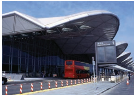
Hong Kong: Zip instant boiling water is installed throughout the stunning Chek Lap Kok Airport.
